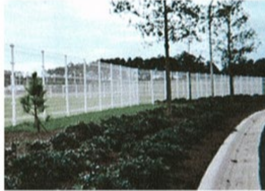
Fence and landscaping along the rail.
